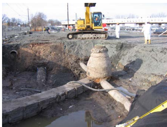
View of exposed sewer manhole during excavation.
