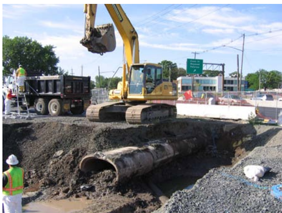
Excavation around elliptical storm drain that runs perpendicular to NJ Route 17.
