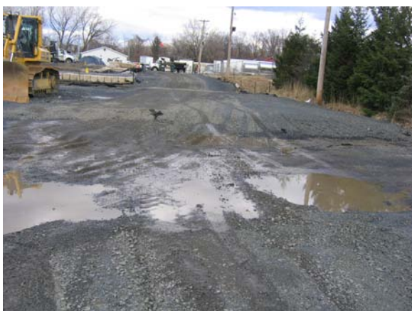
Excavation was backfilled with structural fill, graded and compacted to create haul road.
