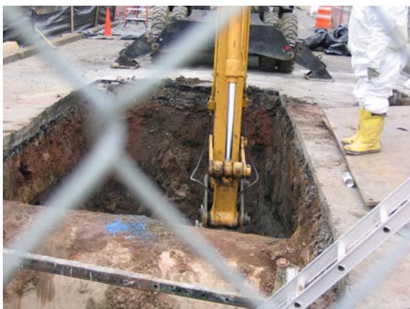
View of area being excavated. Fencing was installed around the excavation.
