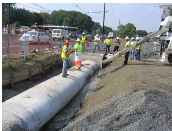
Flowable fill was used for backfilling the excavation around the elliptical pipe.
