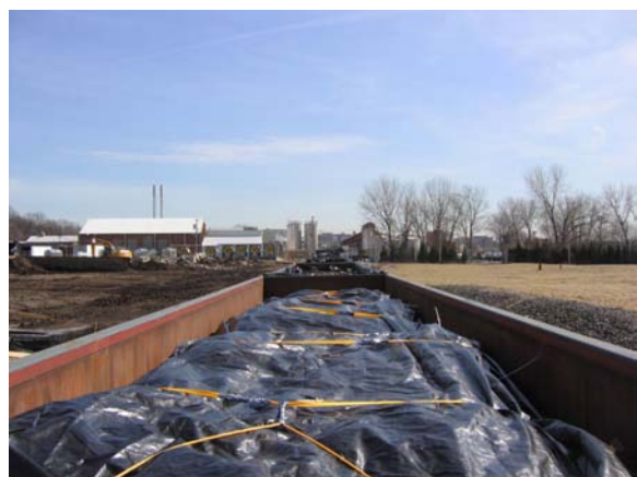
The rail car liners are secured prior to shipment for offsite disposal.
