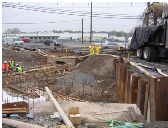
Excavating above a concrete box culvert; collaboration with other construction projects in the area was essential.
