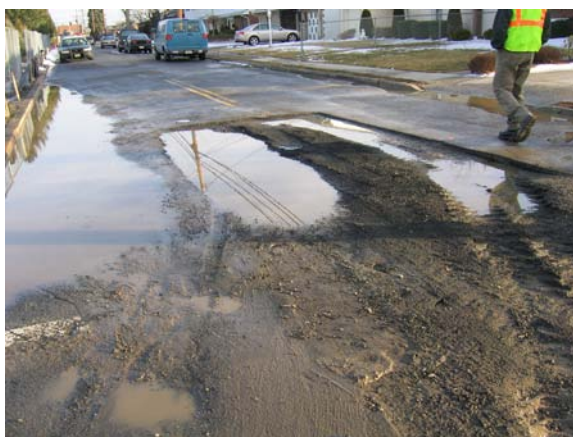
Another view of the excavation after being backfilled with structural fill.
