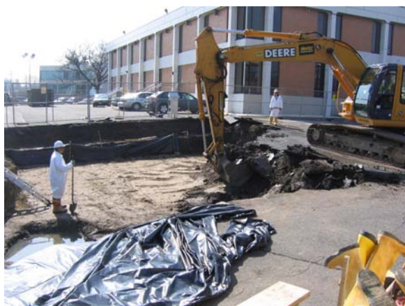
Excavating on the north west side of 113 Essex St. Plastic sheeting was used to cover the contaminated soil.
