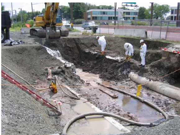
Dewatering of the excavation was performed to remove groundwater.
