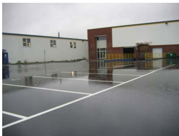
View showing newly paved and striped parking area on northwest of the building addition.
