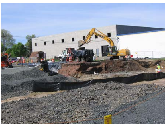
Excavator was used to load the contaminated soil into lined dump trucks for transport to the MISS.
