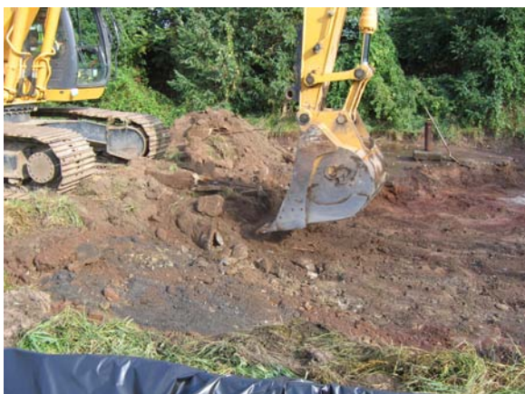
Excavated soil was transported by dump trucks to the soil staging area at the MISS for placement in fabric structure.
