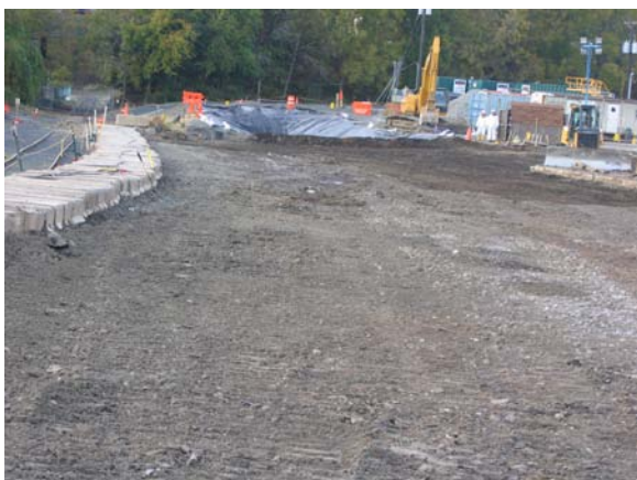
View of graded area along the bulk head for asphalt paving.
