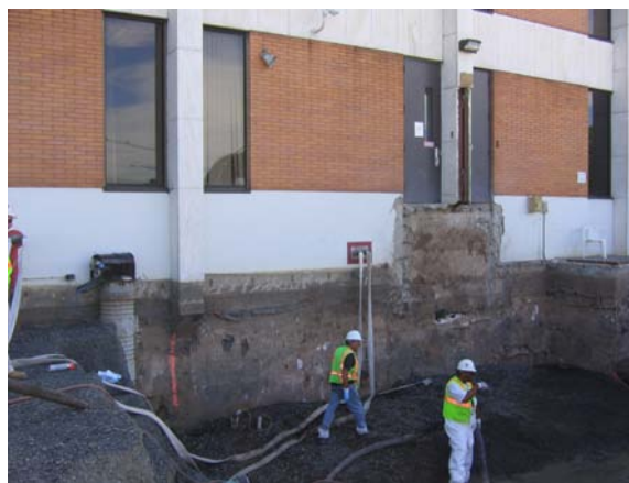
Excavating adjacent to the north side of the building at 113 Essex Street.
