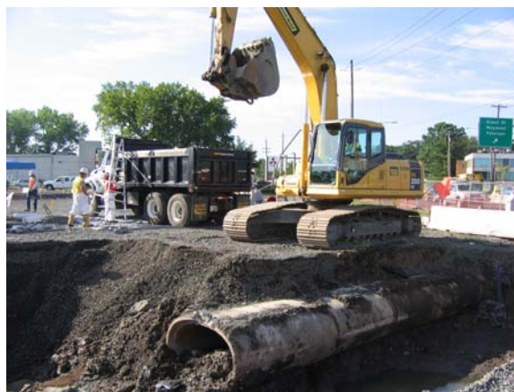
Excavator was used to load contaminated soil into dump truck for transport to the MISS.
