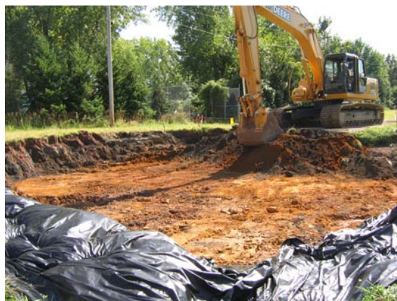
Plastic sheeting was installed at the face of the excavation to separate the excavated areas from contaminated areas.
