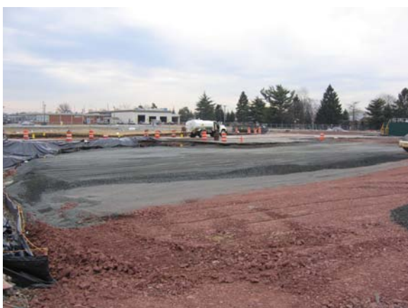
Completed excavation was backfilled with common fill and structural fill.
