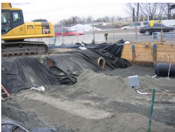
Excavated area adjacent to NJ Route 17 northbound was backfilled with structural fill.
