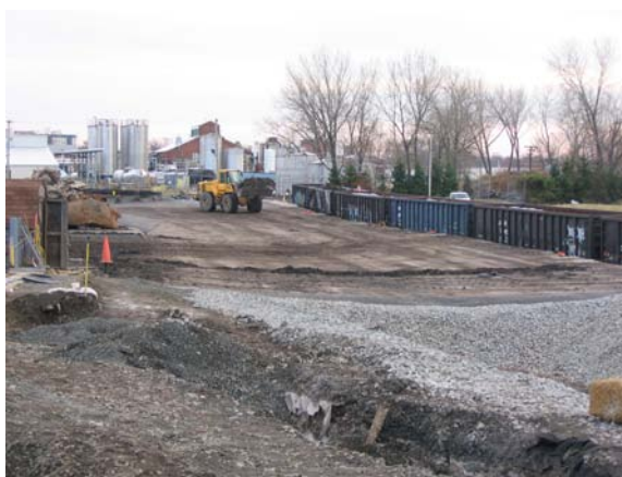
A front end loader on concrete bulkhead placing soil from the fabric structure into lined rail cars for offsite disposal.
