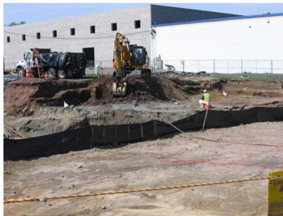
Plastic sheeting was installed at the face of the excavation to separate the excavated areas from contaminated areas.
