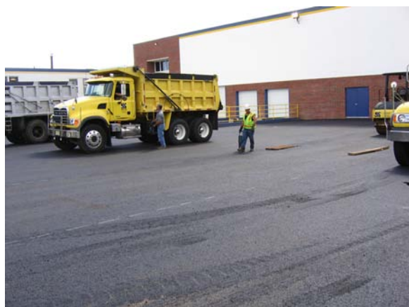
After completion of excavation, building addition was completed and asphalt paving installed.
