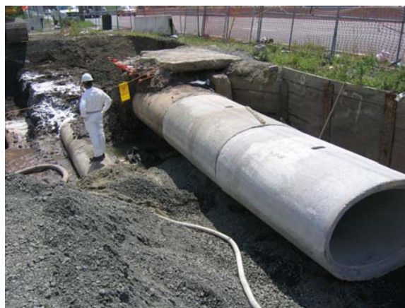
View of the 53 inch by 34 inch elliptical reinforced concrete storm drain adjacent to Route 17 northbound.
