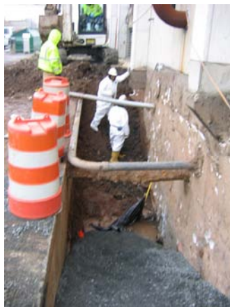
Excavating around utilities on the east side of 113 Essex Street between the building and a concrete box culvert.
