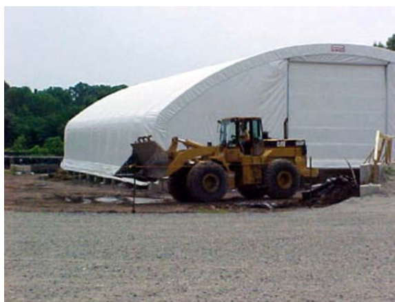
A front end loader is used to transport soil from inside the fabric structure directly to the rail cars.
