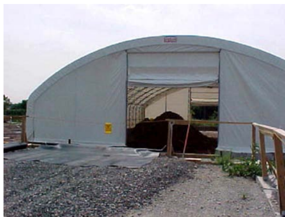
The stockpile of excavated soil from the vicinity properties is stored inside the fabric structure at the MISS prior to the start of load-out activities.
