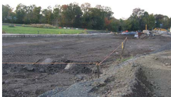
A view of grading activities being performed in the restricted area in preparation for grading activities.
