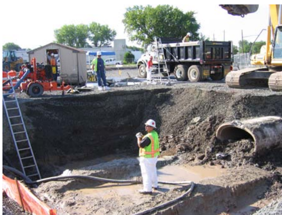
View of deeper excavation within the utility corridor adjacent to Route 17 northbound.
