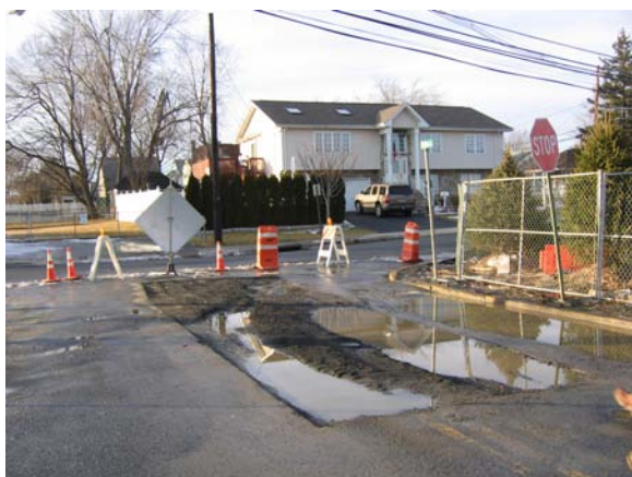
After completion of the water line repairs, the excavated area was backfilled with structural fill.
