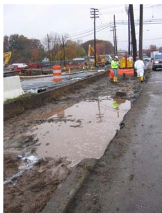
The final status survey crew conducting a radiological survey after completion of the excavation activities.
