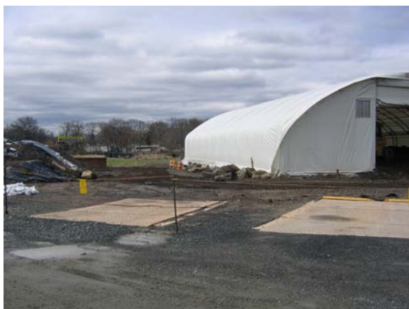
View of the truck dumping area located behind the fabric structure.
