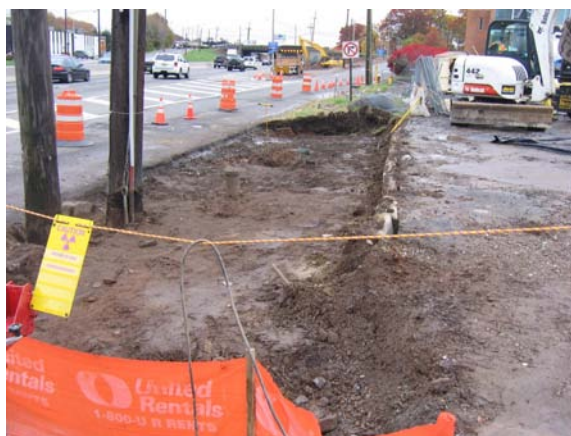
Additional excavation being performed in the NJ Route 17 southbound ROW.
