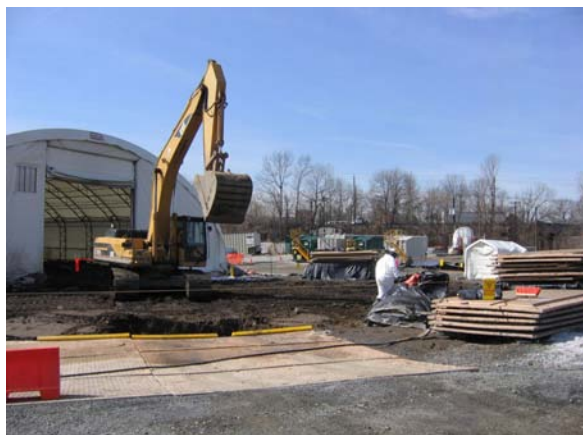
The soil receiving area at the MISS is located behind the fabric structure. An excavator is used to place incoming soil from the vicinity properties into the fabric structure.
