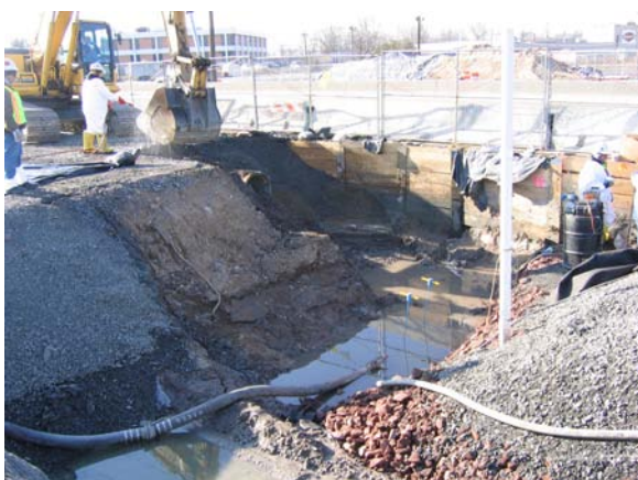
Pumps were used to remove accumulated water in excavation.
