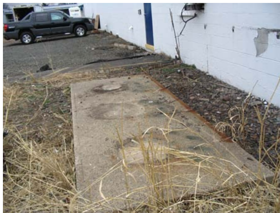
The feeder pole/transformer pad needed to be removed for expansion of building. Area was previously inaccessible.
