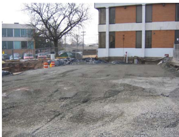
Excavation on the north side of the building at 113 Essex Street was backfilled with structural fill and compacted.
