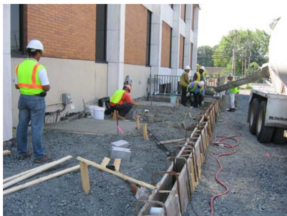
View of concrete form work for restoration activities on the west side of building at 113 Essex Street.
