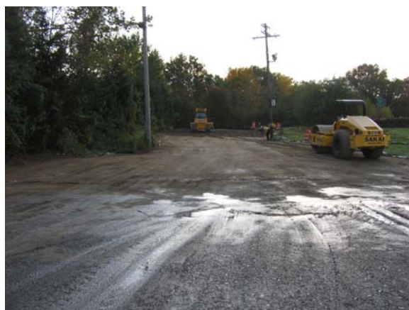
Another view of haul road which will allow the use of much larger capacity dump trucks for soil transport.
