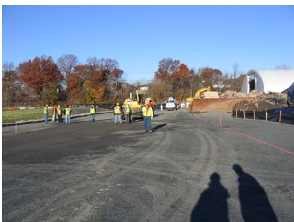
Asphalt installation along the bulk head area.
