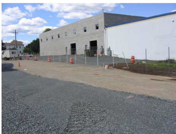
Completion of backfilling the excavation with structural fill.
