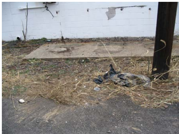
Initial conditions showing the main electrical feeder pole and transformer pad.
