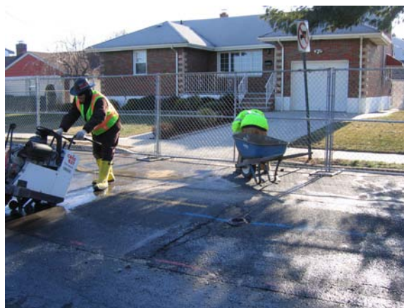
View showing saw cutting of the asphalt pavement on Columbia Lane.
