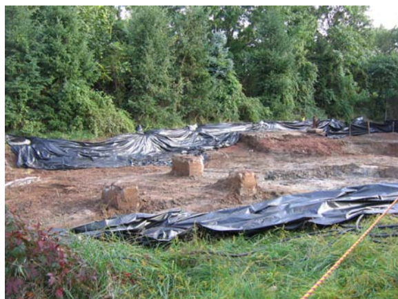
The excavation uncovered old foundations that had to be removed to construct the haul road.
