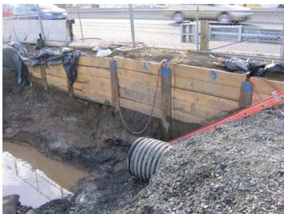
Excavation in utility corridor adjacent to NJ Route 17 northbound.
