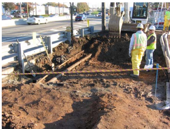
Excavating around a gas line in NJ Route 17 southbound ROW.
