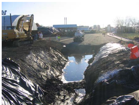
View of asphalt installation and the retention pond.
