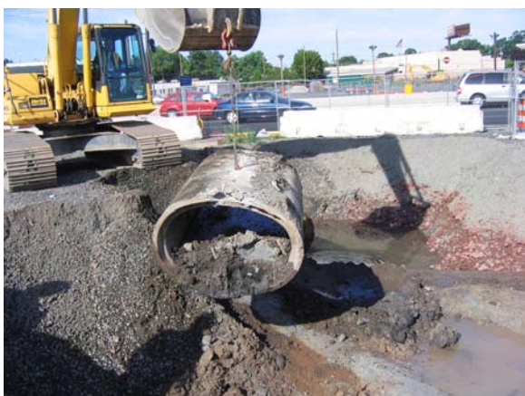
Excavator was used to remove a section of the existing elliptical storm drain.
