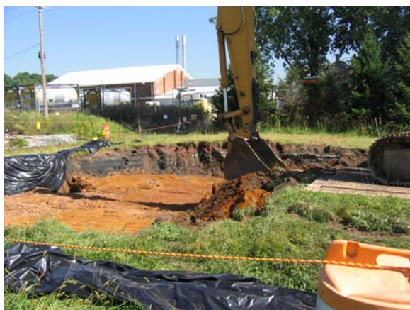
Excavation at the MISS for the construction of the Stepan Haul Road.
