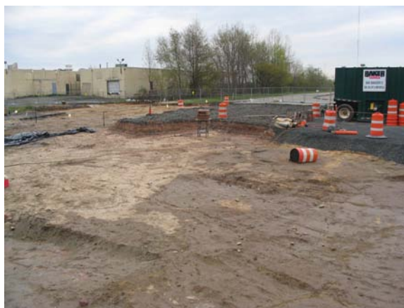
Another view of excavated areas at the NJMVC property.
