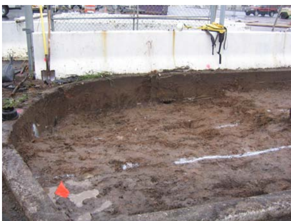
Completed shallow excavation in the NJ Route 17 ROW.
