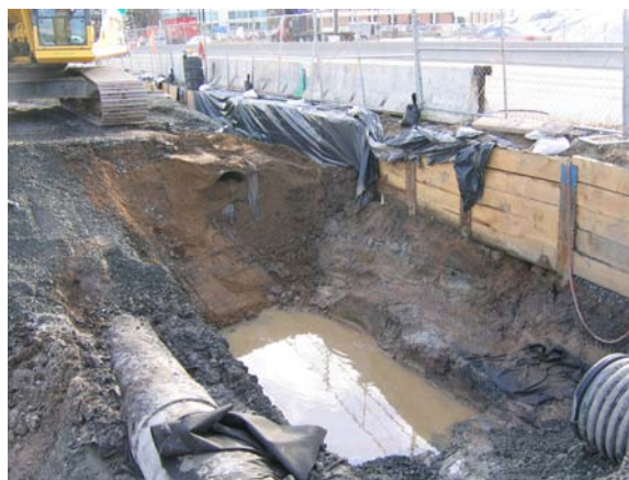
Excavation in the utility corridor exposed high pressure gas main and storm drain.
