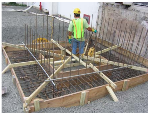
View of concrete form work and reinforcement bars for stair case restoration on the north side of 113 Essex Street.
